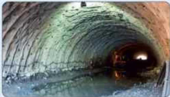
India: Khatpur to Nerchoak Section (Total Length - 6.624 km, Single Tube Bidirectional) Scope: Independent Engineer for Construction Supervision
