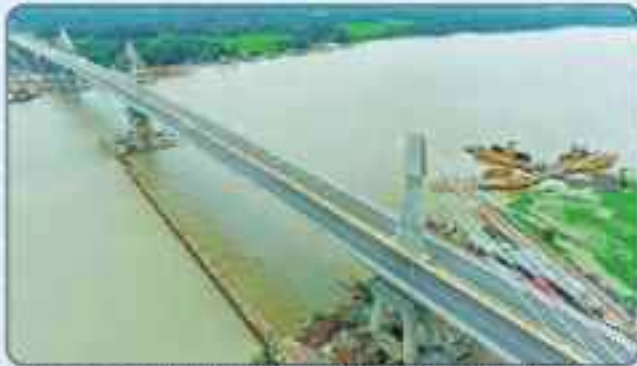
Bangladesh: Faiza Bridge (4 Lane, 1.47 km - Extradosed), KfAED funded Scope: Detailed Design, Bid Management & Construction Supervision
