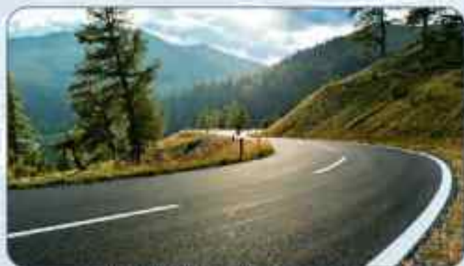
India: NH-229 (Neshpu - Hsi), Arunachal Pradesh Scope: Lender's Independent Engineer
