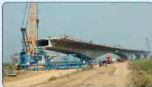
India: Bantiyapur Bridge (4 Lane, 5.55 km) Scope: Independent Engineer for Construction Supervision
