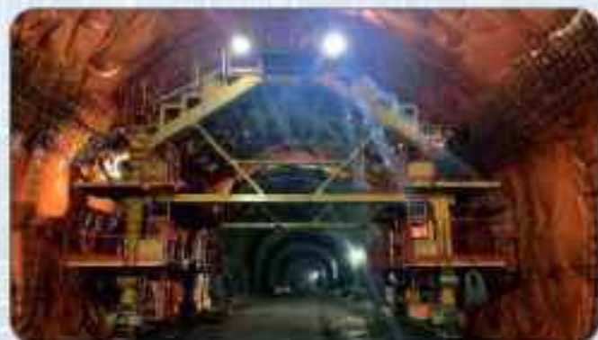
India: Z-Moh Tunnel (Main Tunnel Length - 6.412 km, Single Tube Bi-Directional) Scope: Independent Engineer for Construction Supervision
