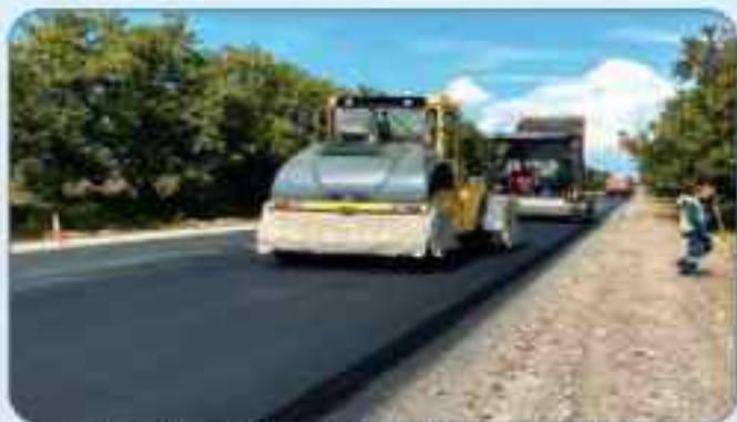
Moravia Road Rehabilitation Project-IV (83 km), EBRD funded Scope: Construction Supervision under FIDIC Conditions of Contract
