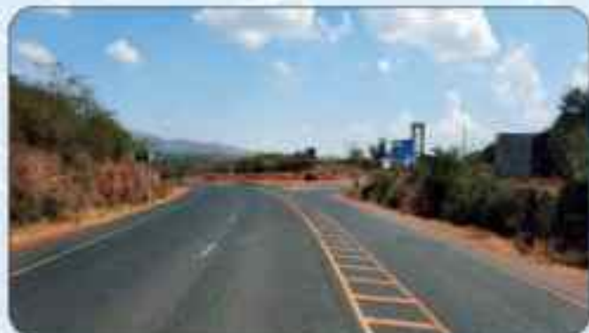
Kenya: Nairobi-Nakuru-Mau (A104 near AB) Highway, World Bank funded One of the largest PPP Projects of Africa Scope: Technical Feasibility and Transaction Advisory
