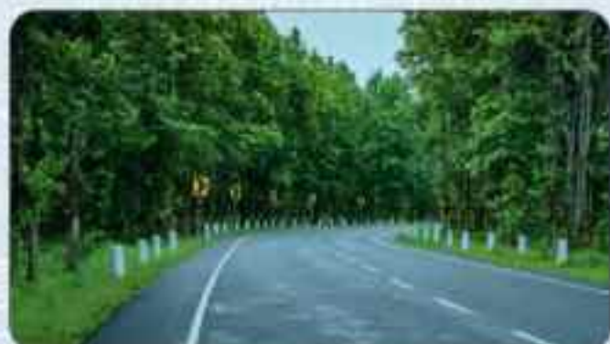
India: Assam State Roads Project (220 km), World Bank funded Scope: Road Safety Audit, Detailed Design for Blackspot Improvements, Capacity Building including Development of Road Safety Investment Framework
