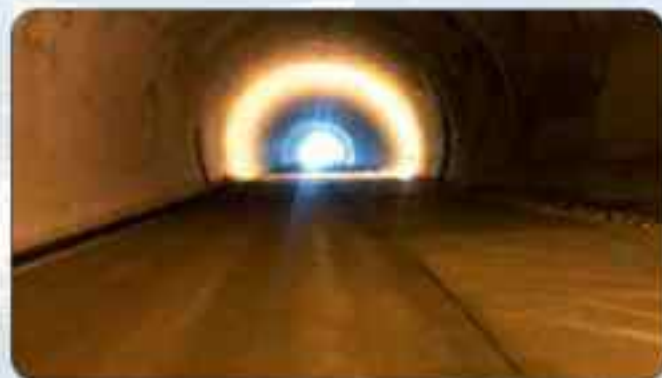
India: NH-21, Pandoh Bypass, Takai Section (Total Length 14.983 km, Single & Twin Tube Tunnels) Scope: Independent Engineer / Construction Supervision
