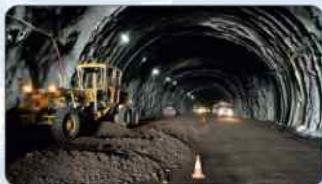
India: Delhi-Vadodra Access Controlled Expressway Package 10 (Total Length - 3.65 km, Twin Tube) Scope: Authority's Engineer for Construction Supervision
