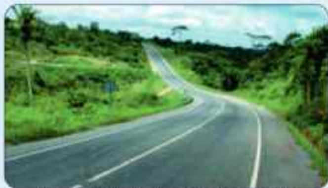
Ghana: Fufuleh-Serele Road Project (147.50 kms, AfDB funded) Scope: Construction Supervision
