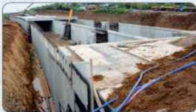
India: Gurgaon Expressway (Total Length - 3.9 km) Scope: Authority's Engineer for Construction Supervision
