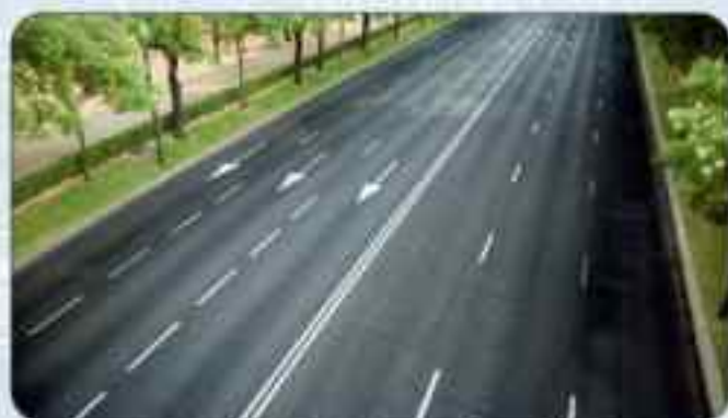
India: NH-8, Surat-Dahisar Section (6 Lane, 239 km) Scope: Independent Engineer / Construction Supervision
