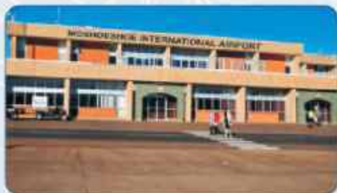
Lesotho: Mosheshwe I International Airport Scope: Economic Feasibility, Detailed Engineering Design & Airport Master Planning
