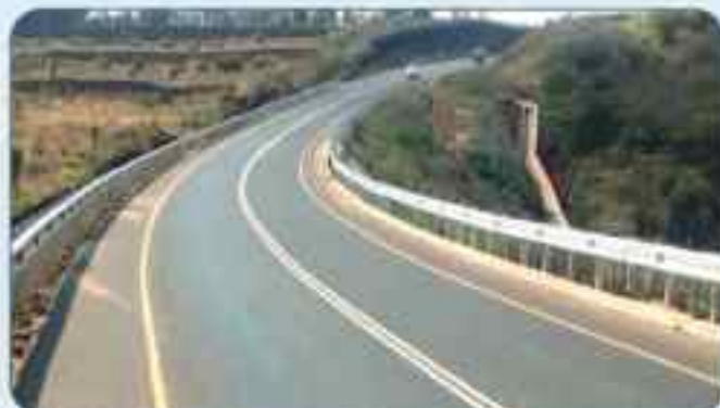
Tanzania: Multinational Arusha-Hellio / Taveta-Voi Road Corridor Development Project (2 Lane, 56.5km), AfDB funded Scope: Road Safety Audit, Road Safety Education & Campaign & Capacity Building
