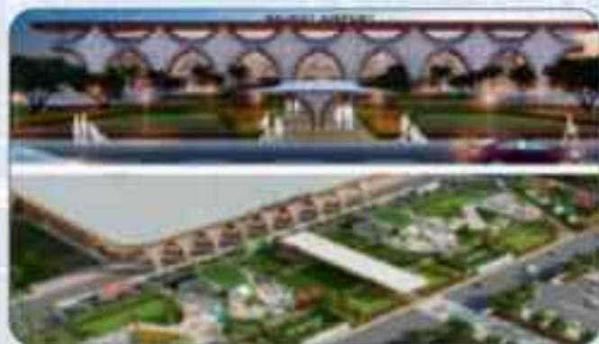
India: New Greenfield Airport at Hirasar, Rajkot Scope: Project Management Consultancy Services
