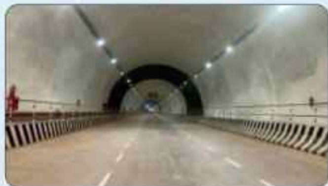
India: NH-47, Vadakkancherry-Thressur Section (Total Length - 1.925 km, Twin Tube) Scope: Independent Engineer for Construction Supervision
