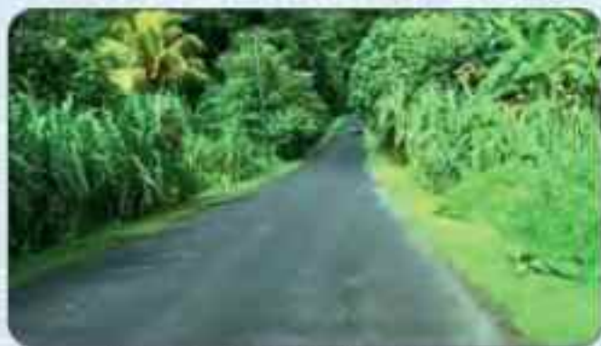
Microesia: Climate Resilience Improvement Works for identified Road Network Assets, World Bank Funded Scope: Detailed Design and Construction Supervision
