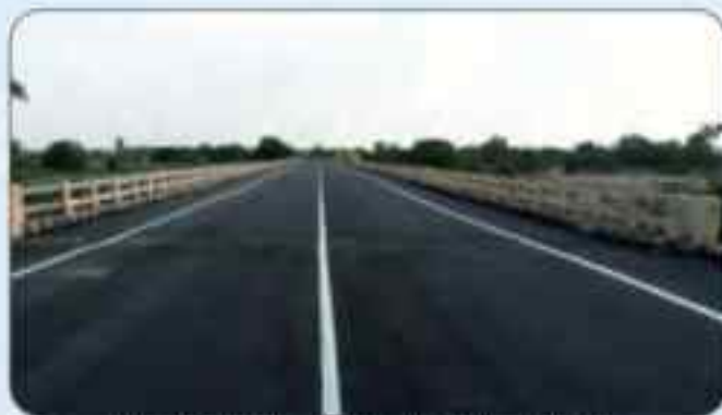
India: NH-98, Anisabad Aurangabad (narharganj) Section (154.625 km), World Bank funded Scope: Construction Supervision under FIDIC Conditions of Contract
