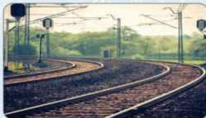
India: Elevated Railway Line in Kurukshetra (Length: 5.18 km) Scope: Survey & Design
